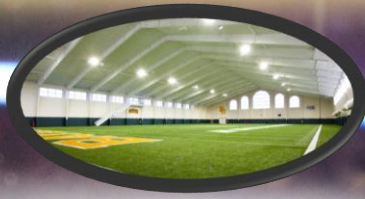
Allison Indoor Facility
